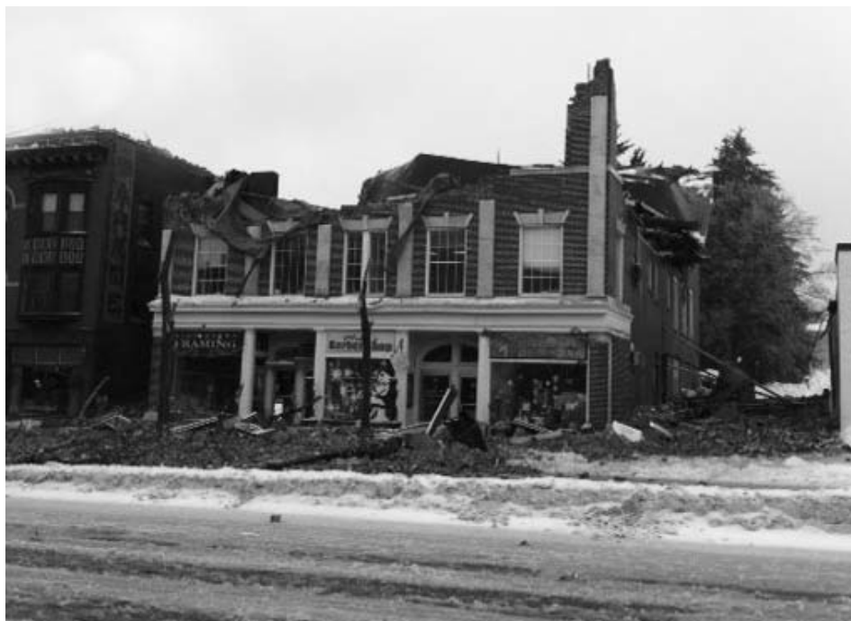
Guilmartin, DiPiro & Sokolowski, LLC's building at 505 Main St. in Middletown, which collapsed under the weight of snow and ice on February 2. Only two stories of the formerly three-story building remain.
